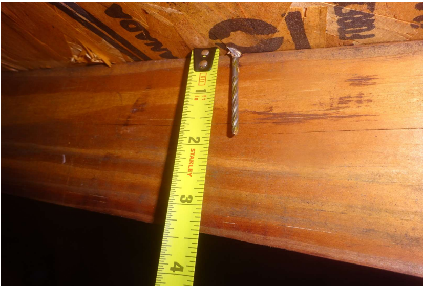
8d nails verified
